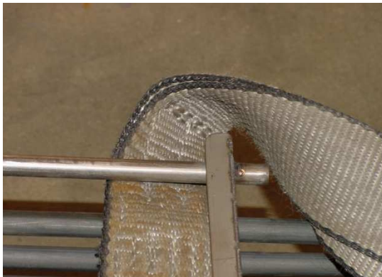
Figure 3 - Install Lifting strap between element bundle and support bracket. Do not entwine straps between elements. Place second strap around terminal enclosure.
