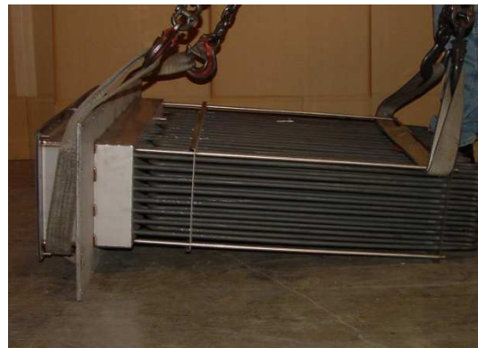
Figure 3 - Install Lifting strap between element bundle and support bracket. Do not entwine straps between elements. Place second strap around terminal enclosure.
